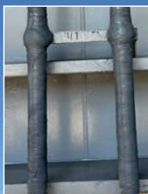
Inset pictures: various gas and water pipes protected with the modified Steelcoat 100/400™ System
