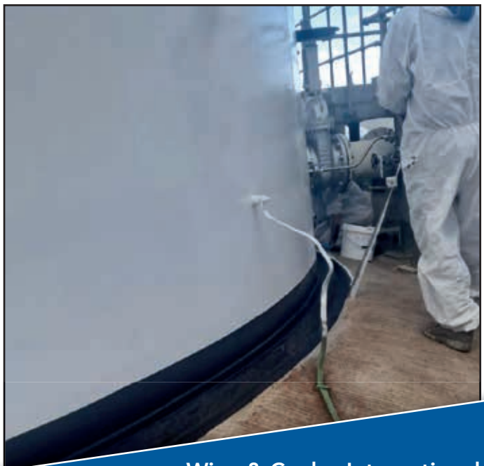
The Viscotaq™ Chime Sealing System applied to the fuel storage tank.
