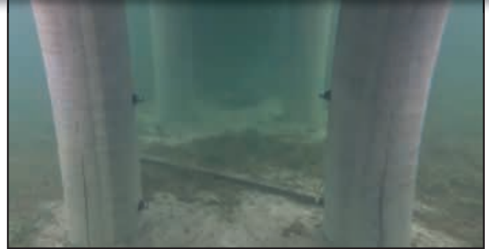
Underwater view of the completed SeaShield 400™ System.
