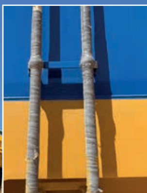
Inset pictures: various gas and water pipes protected with the modified Steelcoat 100/400™ System
