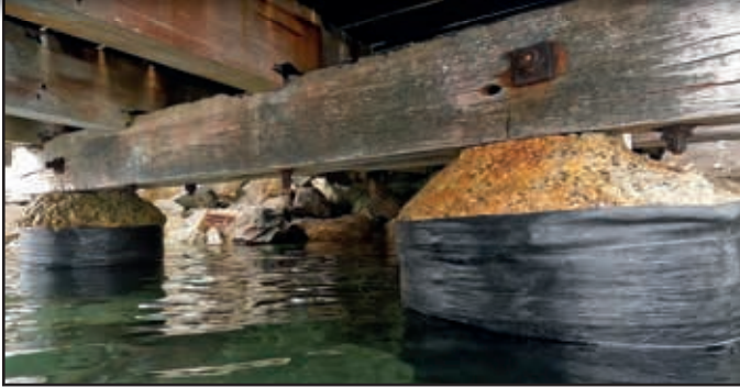
The completed SeaShield 70™ System.
