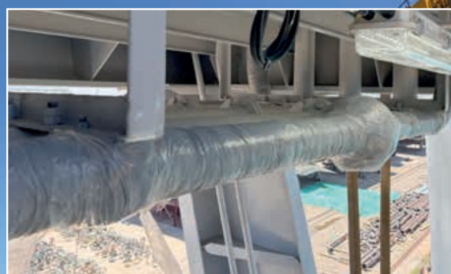
Inset pictures: various gas and water pipes protected with the modified Steelcoat 100/400™ System
